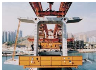
Rambler Channel Rail Bridge
