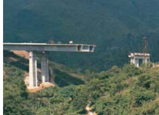
Liu To Bridge
