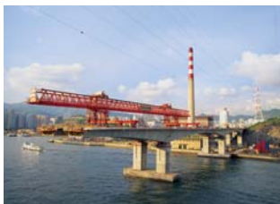
Rambler Channel Bridge
