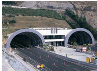
Cheung Tsing Tunnel
