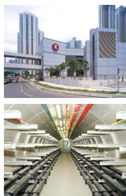
top MTR Hang Hau Station bottom Tsz Wan Shan Cable Tunnel
