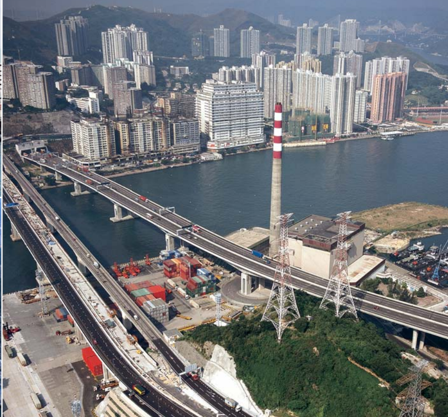
Rambler Channel Bridge
